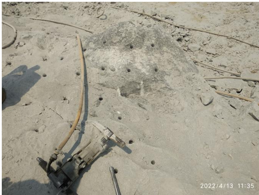
Figure 5. Drilling pattern of holes (20-30 cm spacing)
