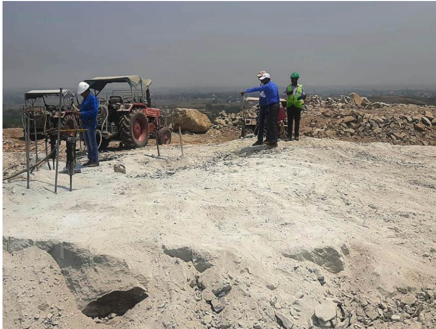
Figure 4. Use of 32 mm diameter Jack Hammer Drilling Machine for drilling of holes
