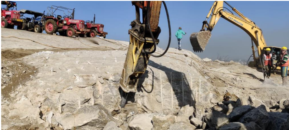
Figure 7. Use of Hydraulic Rock Breakers to break the cracks generated by the non-explosive agent
