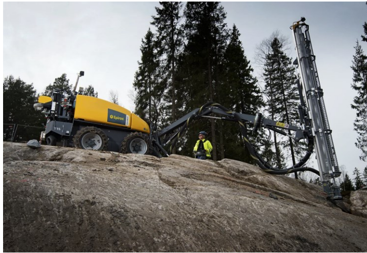
Figure 4 Construction of boreholes to stabilize the slope (Epiroc, 2024b)
