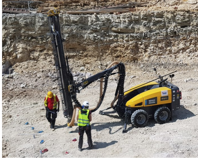
Figure 3 Atlas Copco FlexiRoc T15 self-propelled drill machine on worksite
