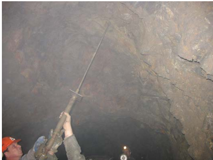
Figure 3 - Mounting of the fiberglass rockbolt into the excavation drift side wall
