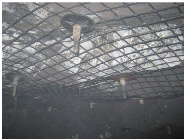
Figure 5 - Rockbolts mounted in combination with steel mesh
