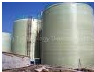
Figure 4 - GRP storage tanks
