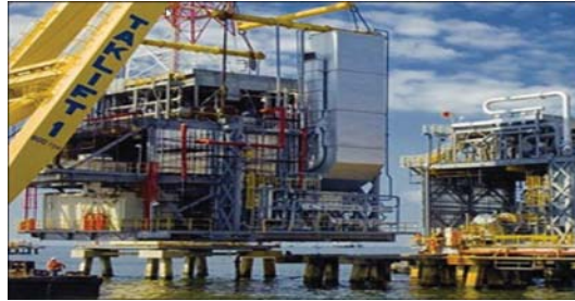
Figure 11 - Replacing of steel installations with fiberglass pipes in Maracaibo bay
