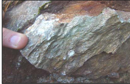
Figure 1 Prvonek dam, gneiss detail (photo D. Milovanović)
