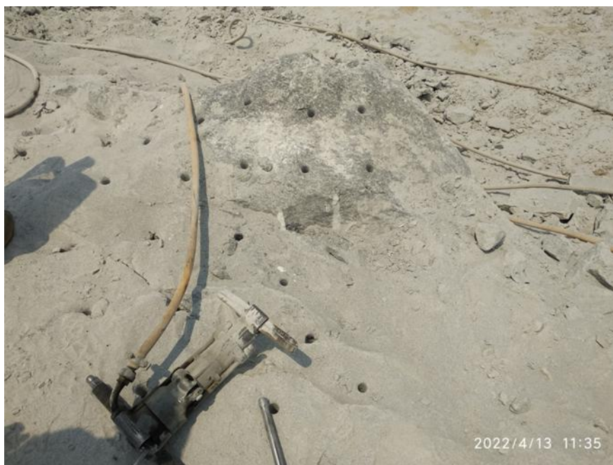
Figure 5. Drilling pattern of holes (20-30 cm spacing)
