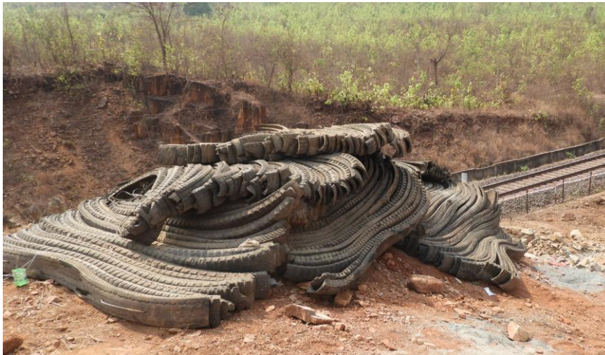
Figure 12. Muffling/covering of blasting patch using blasting mats
