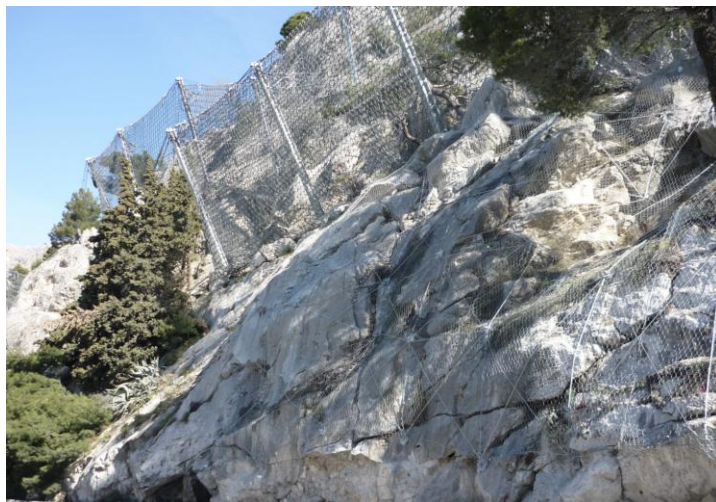
Figure 5 Protective net-protection against the rock fall (Geotech, 2024)
