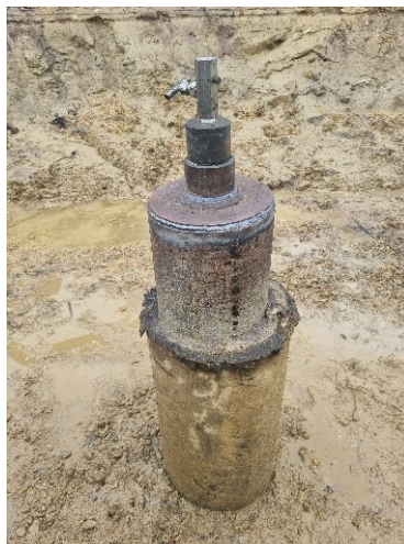
Figure 3 An abandoned well with a cover cap
