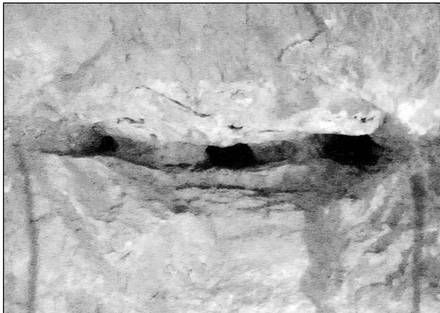
Figure 3 Line cut after blasting
